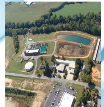
Mauldin Road Water Treatment Plant
